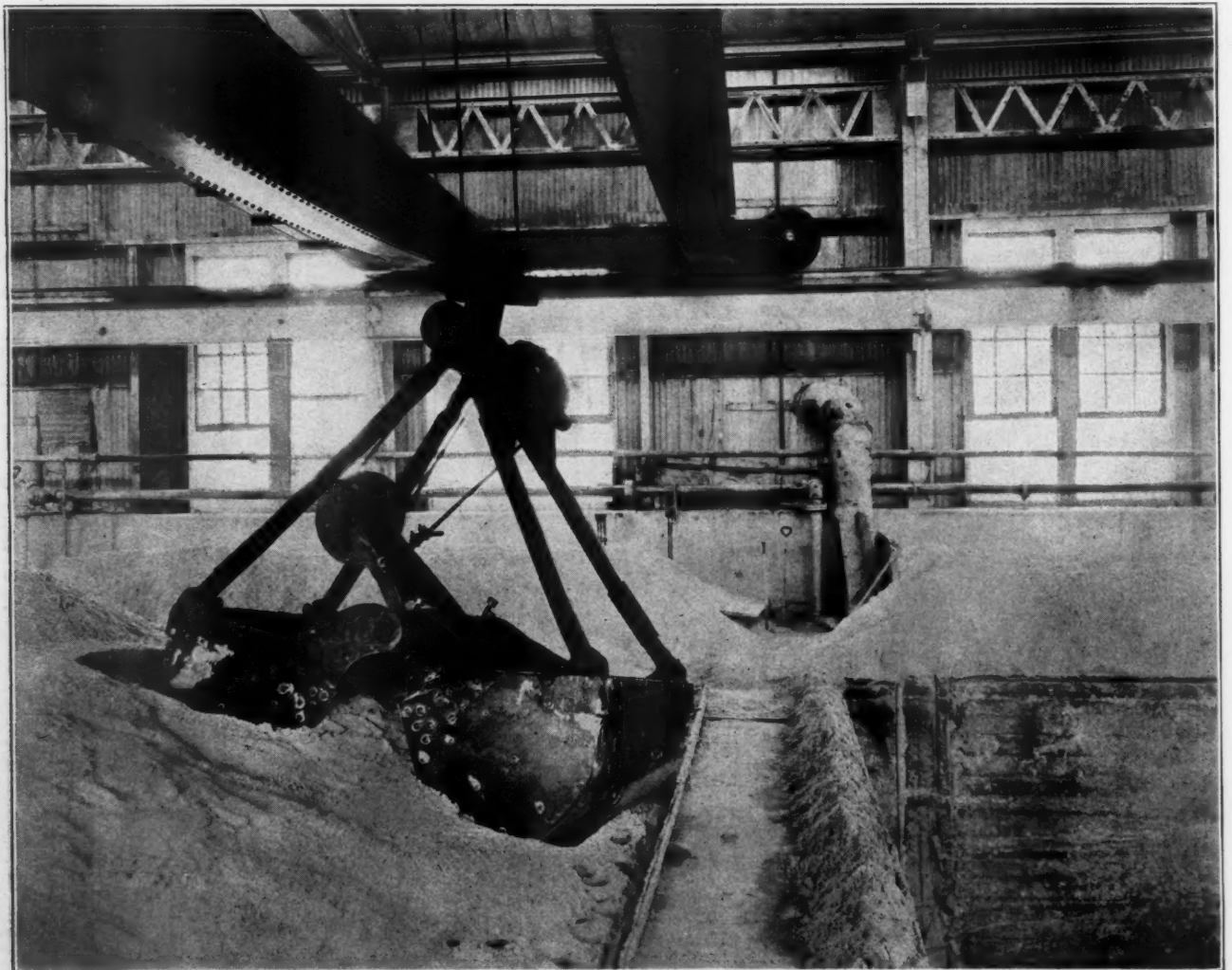
Removing Sand From a Drain Bin
